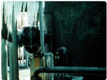
Here, a dock door was left open overnight. The extreme temperature caused freezing of the overhead water supply to the hydrant. This resulted in considerable leakage from the pipe.
