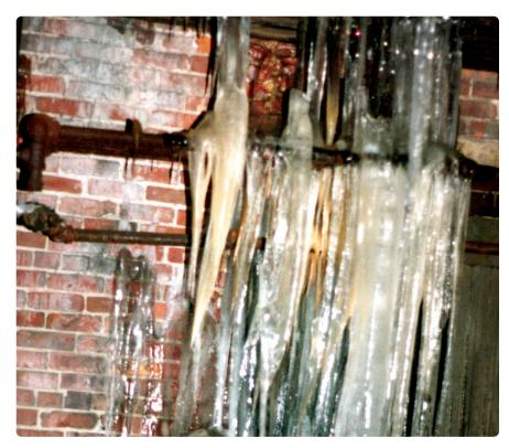
The plan to increase minimum heat in this idle building was far from adequate and resulted in extensive freeze damage.
